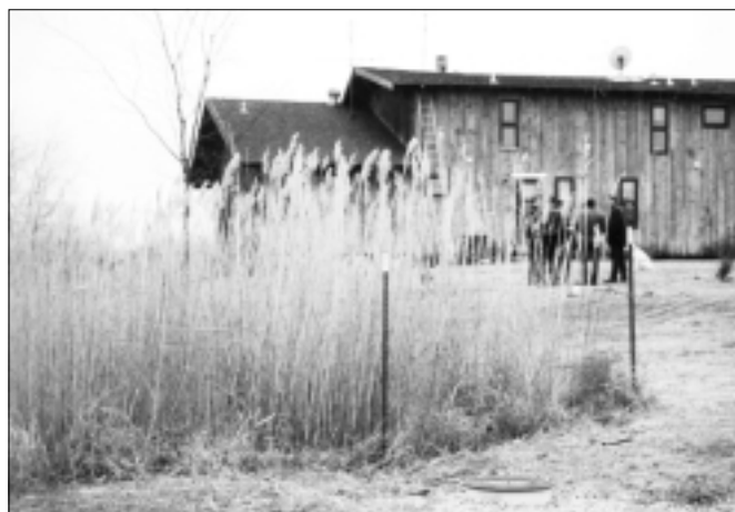
The Carlson Site system with established common reed ( Phragmites australis ). A rock-plant filter can be an attractive component of a residential landscape.
