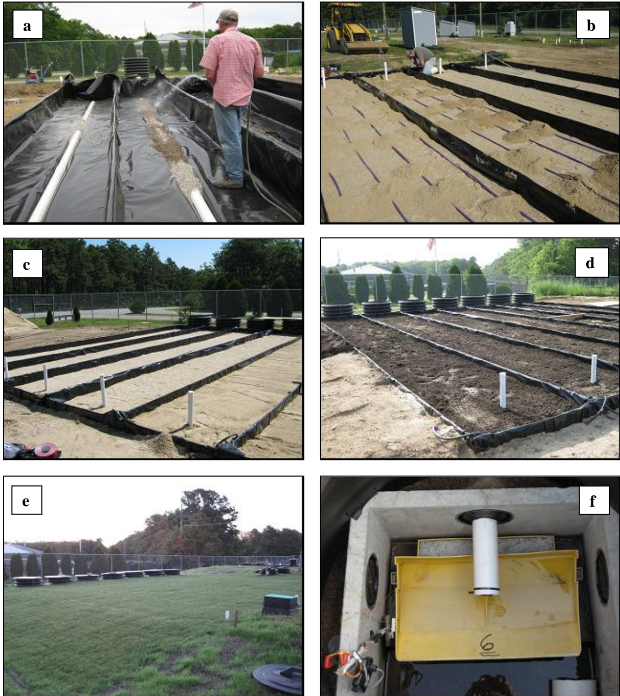
Figure 2. a.) Cell liner installed with sloped sides (toward center drain) and washed peastone around distally-sloped center drain; b.) drip tubing placed within each cell, 16 inches on center, and outer tubing lengths six inches from liner sides; c.) drip tubing with two inches of sand cover before loam cover; d.) two inches of loam spread and raked into sand cover to provide sand-loam transition; e.) finished cells with sod in place; f.) tipper tray inside riser receiving bottom drain pipe—note magnetic-switch operated data logger for recording approximate volume by number of tips.
