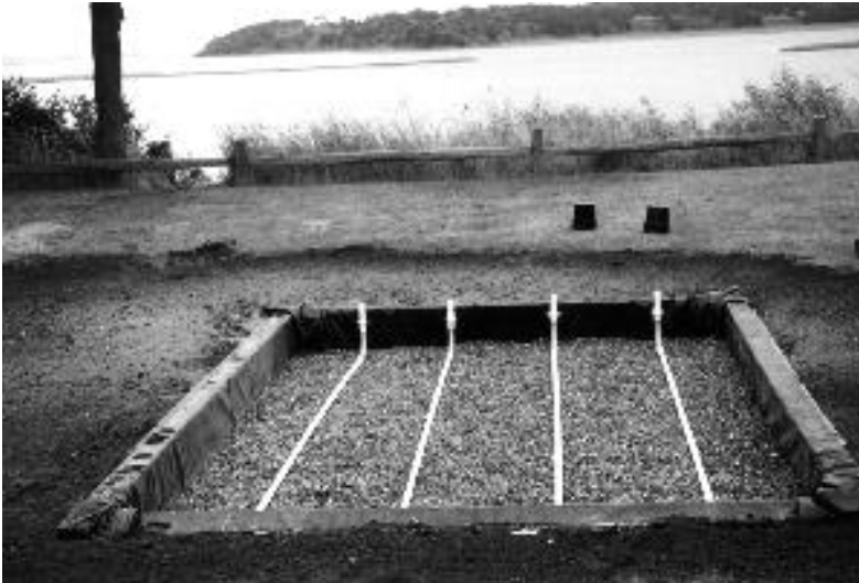
Figure 4. Pressure distribution system of a RSF in Orleans, Ma. prior to the installation of protective caps for the spray orifices, peastone, filter fabric, and a top coating of bark mulch. The finished sand filter is only slightly above the surrounding grade.
